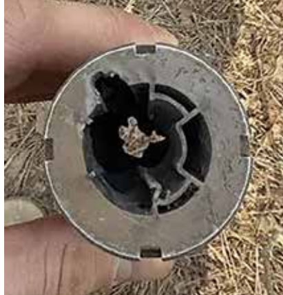
One of the vulnerable structural components: a broken fire and sound suppressor.
